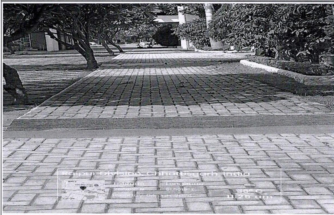
Signage Including Tactile Path, Lights, Display Boards and Signposts
